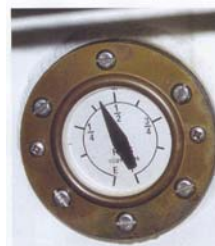
above Removing a tank gauge could allow access for a circulation pipe.
